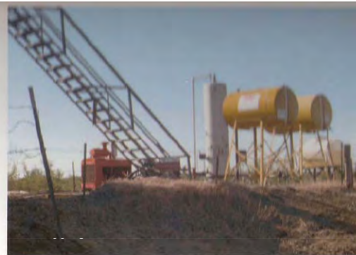
Photo No. 2 – Patrick Welder Tank Battery
